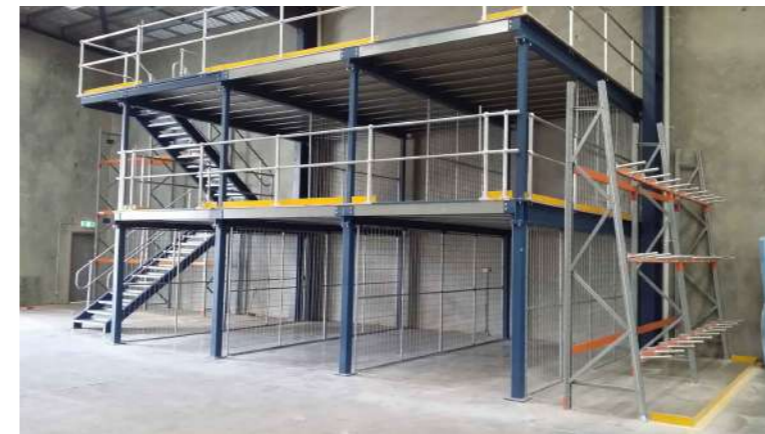
- Light Steel Structure
